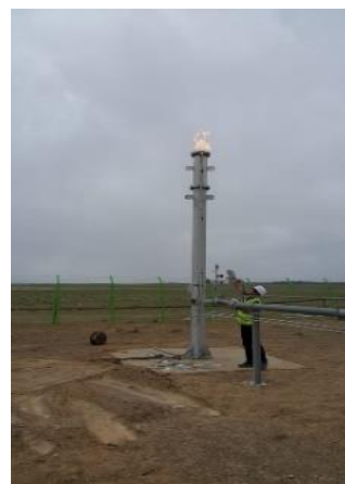
Fig.5 Pilot plant in Tavan Tolgoi: Methane combustion
